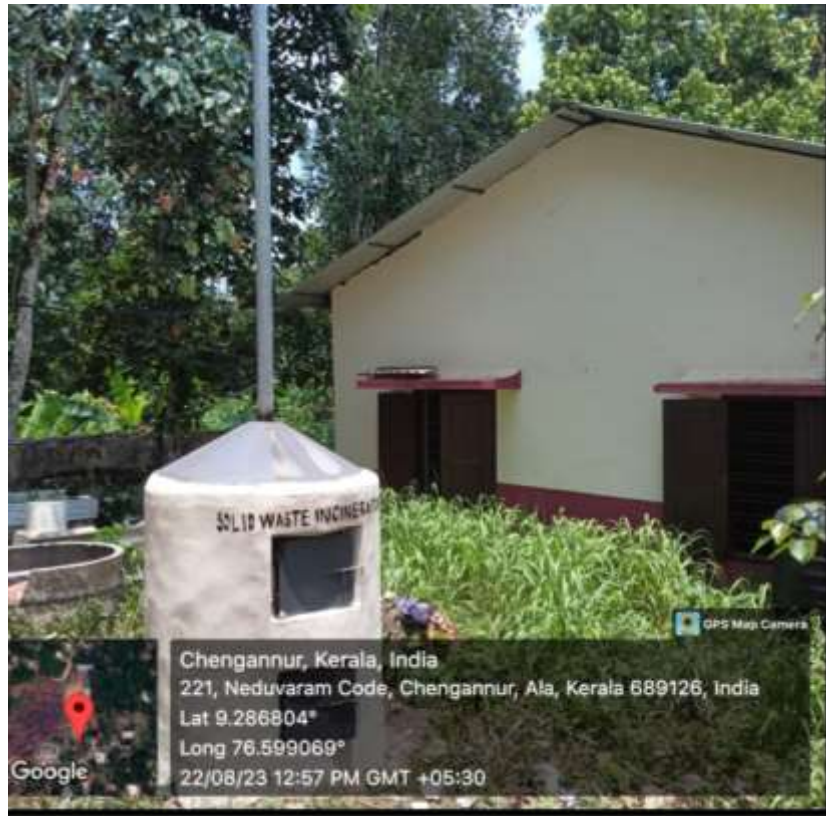
Solid Waste Incinerator
