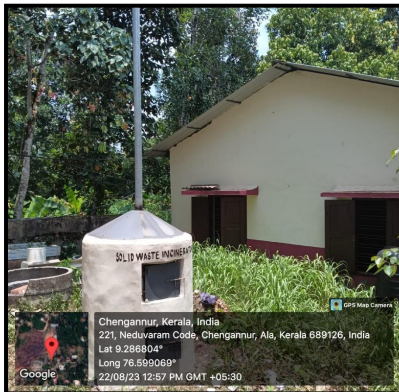
Solid Waste Incinerator installed at the campus
